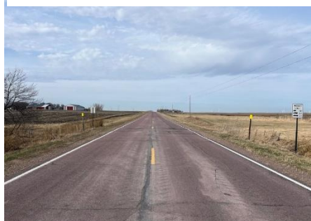
Bridge 93293 – Looking North
