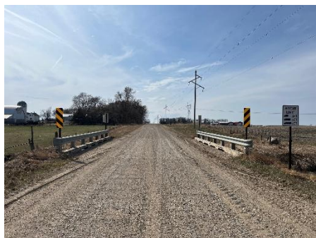
Bridge 32503 – looking west
